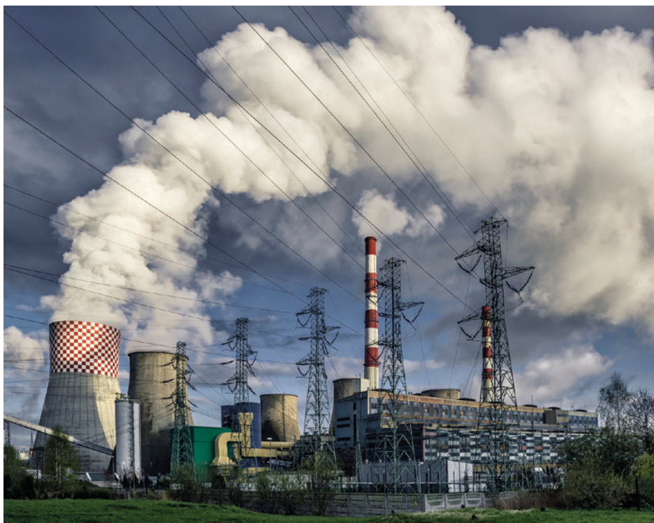
FIGURE 2.1.1 Most power plants use thermal energy to produce steam. That steam does work turning turbines, which generate electricity.
