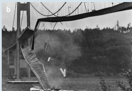
FIGURE 10.4.9 Original photos of the Tacoma bridge collapse. (a) The bridge oscillating due to resonance between the wind gusts and the natural frequency of the bridge. (b) The bridge after collapse.
