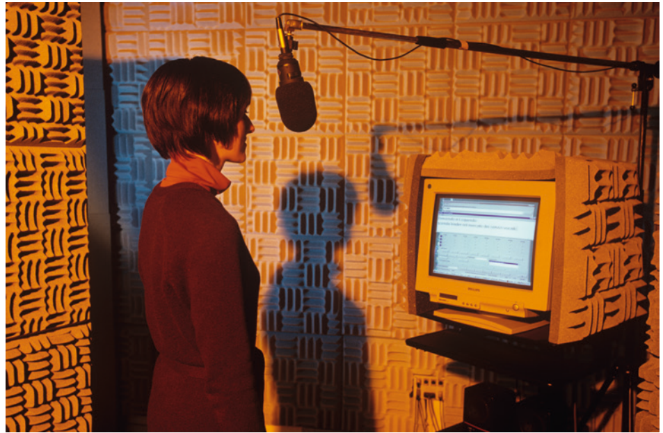
FIGURE 10.6.7 In a recording studio foam is used to absorb sound and corrugations are used to reduce unwanted reflections.
